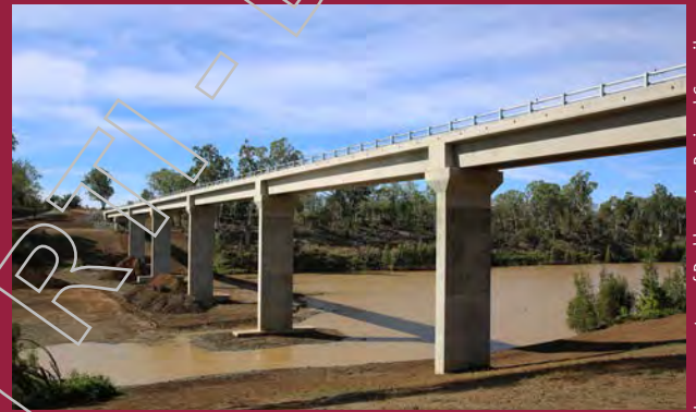
Image courtesy of Rockhampton Regional Council
